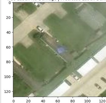
True Label: No Damage | Predicted Label: Damage
